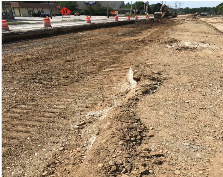
Excavated to subgrade from EB Forest Home.
