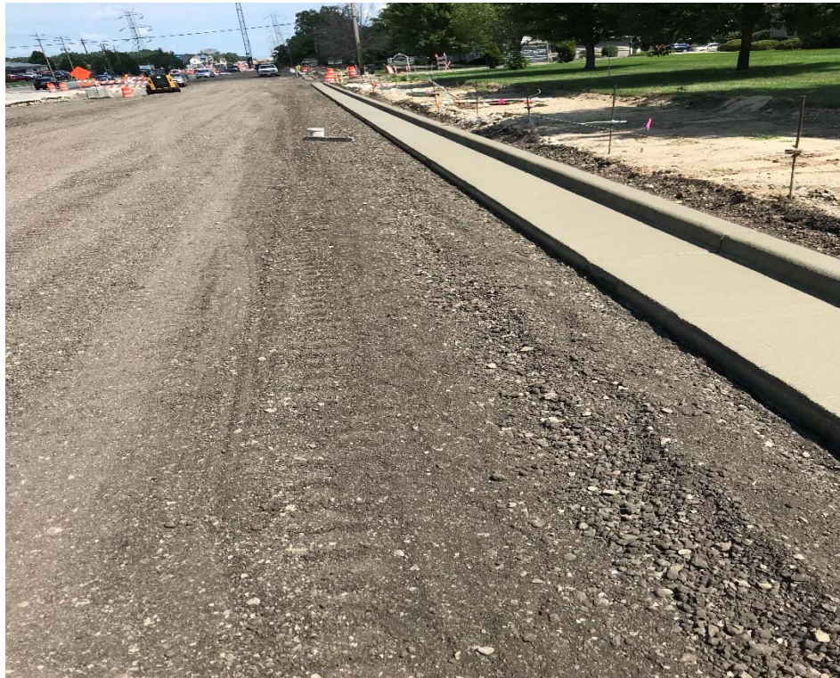
Pouring concrete curb from Kay Parkway to South Limit.
