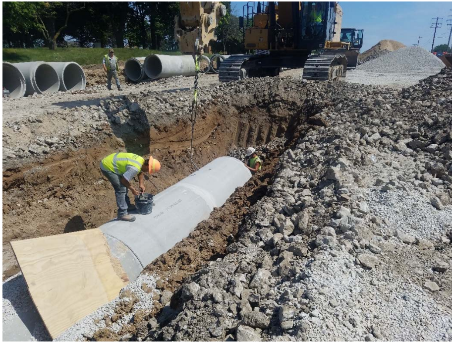
Placement of Storm Sewer Trunkline along Forest Home Ave.
