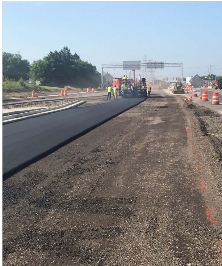
Crews paving the lower lift of asphaltic pavement at the I-43 NB on-ramps.
