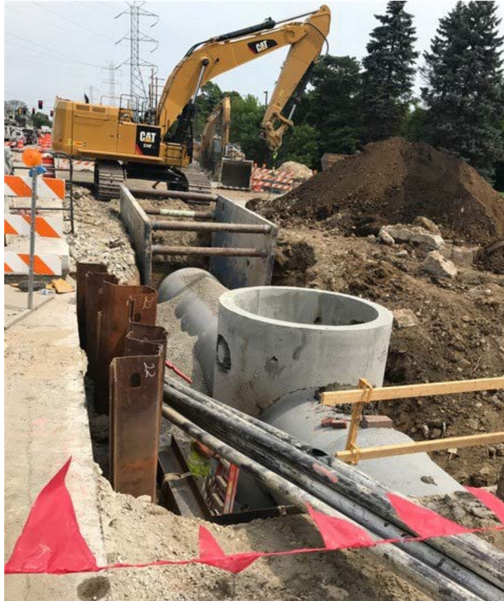
Storm sewer trunkline and manhole north of Whitnall Park Creek box culvert.
