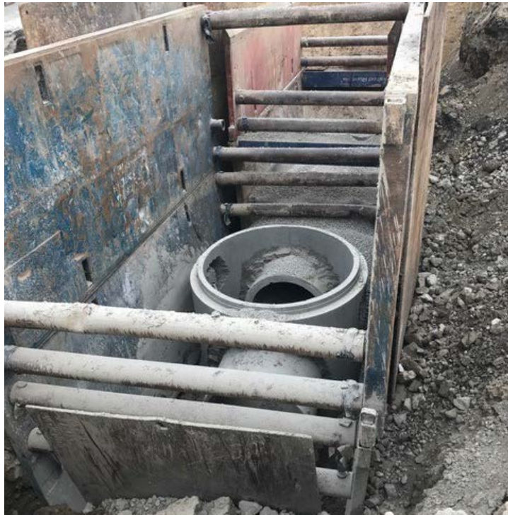
Storm sewer trunkline and manhole east side of Hwy 100, just north of Abbott Ave.
