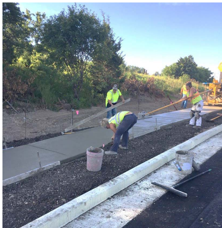
Crews placing concrete sidewalk along the east side of Hwy 100 north of Edgerton Ave.
