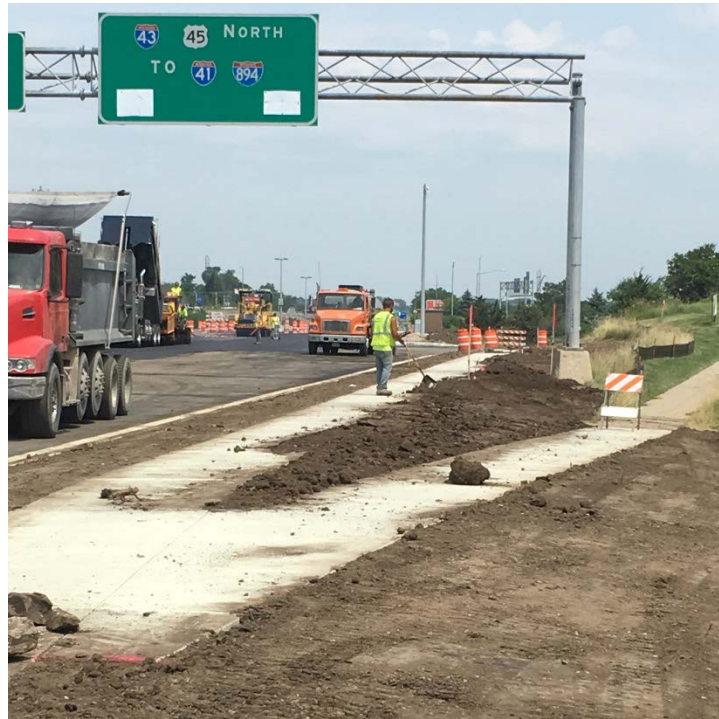
Crews placing topsoil along the sidewalk and curb at the Hwy 100 to I-43 NB on-ramp.
