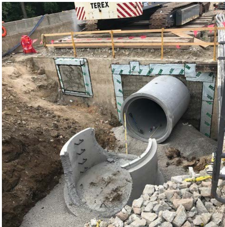
Storm sewer trunkline and manhole at north side of Whitnall Park Creek box culvert.
